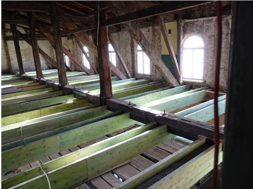
**Relief of the dilapidated beams by side timbers.**
